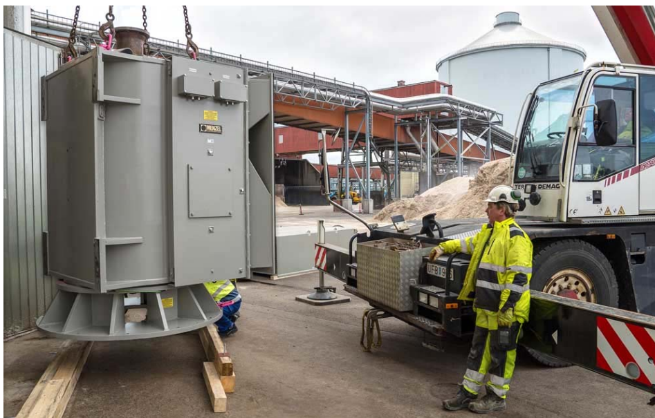
Illustration: Menzel has customized a motor for vertical installation with a welded foot mounting so that the sugar centrifuge can be restarted
